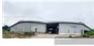
FRONT VIEW OF THE BUILDING
